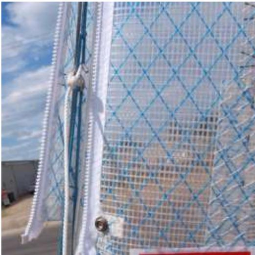
Pull the zip runner the remainder of the way down and close the webbing with the press stud.
